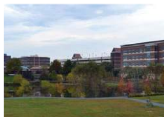
Valley Health Hospital 100+ MOBOTIX Cameras, U.S.A.
