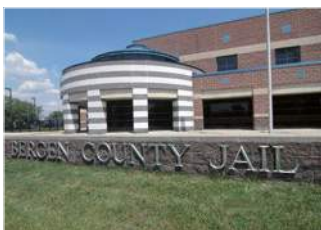
Bergen County Jail 820 MOBOTIX Cameras, U.S.A.
