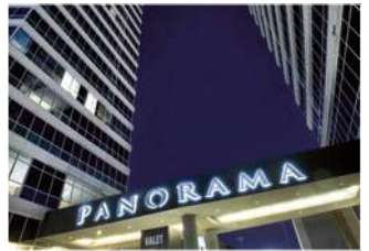
Panorama Towers 137 MOBOTIX Cameras, U.S.A.
